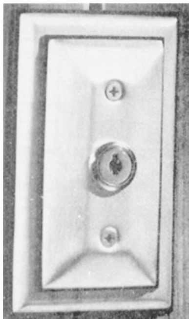
Figure 7.23 A key-operated delayed entry control.
